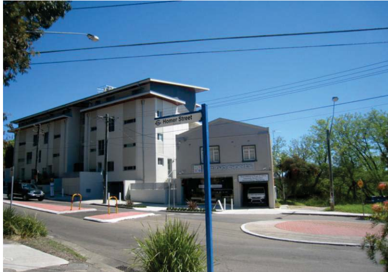
Photo of site at 25-33 Homer Street and subject site
